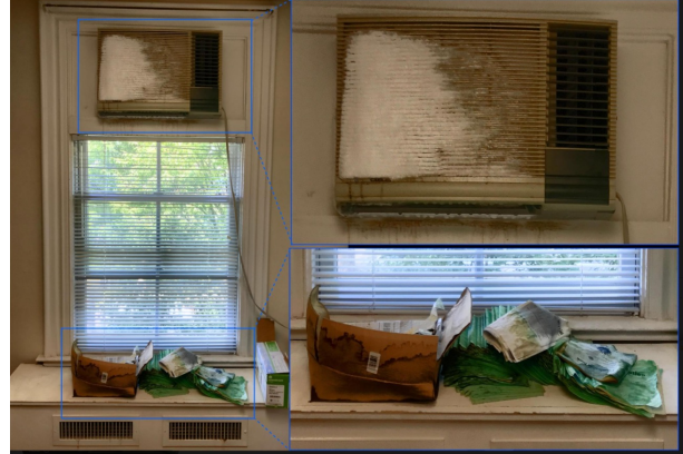
Source: Faculty photo of office, Building P (2108G). September 2, 2021.
